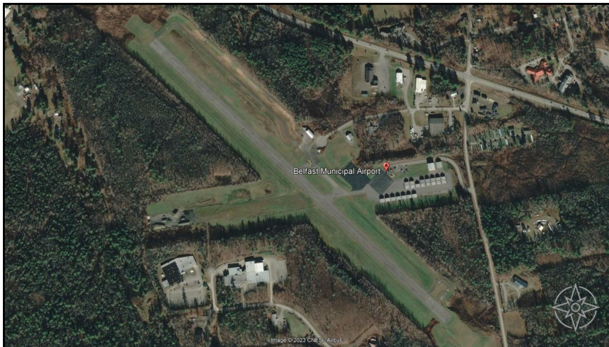
Figure A-1: Belfast Municipal Airport
